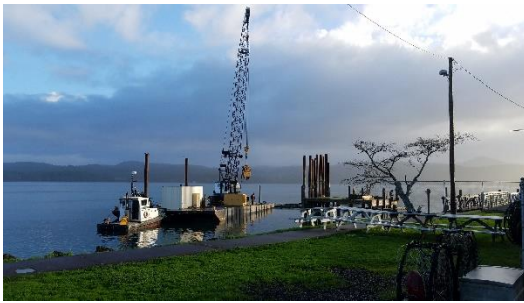
Removing Pilings
